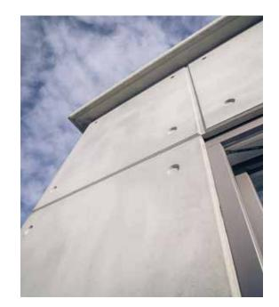
The primary goal was the construction of a building that was completely free from insulation materials based on crude oil. In addition to this was the aim of gaining experience with textile-reinforced concrete during the manufacturing of precast concrete components and their handling in the prefabricated parts facility.
